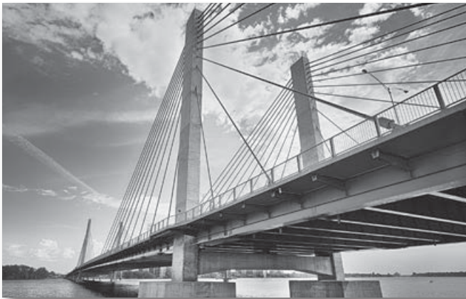
Highway 25 Bridge, Montreal, QC
