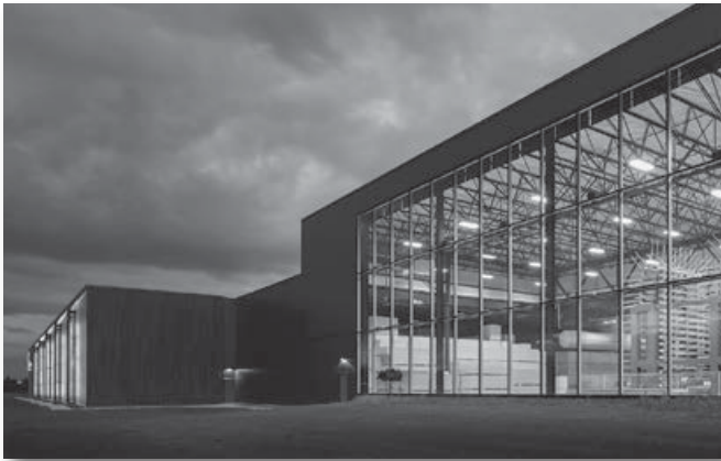
Soprema Plant, Drummondville, QC
